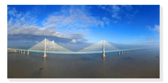
The Shanghai-Suzhou-Nantong Yangtze River Bridge – the world's first cable-stayed bridge with a span of over 1,000 m for both highways and railways
